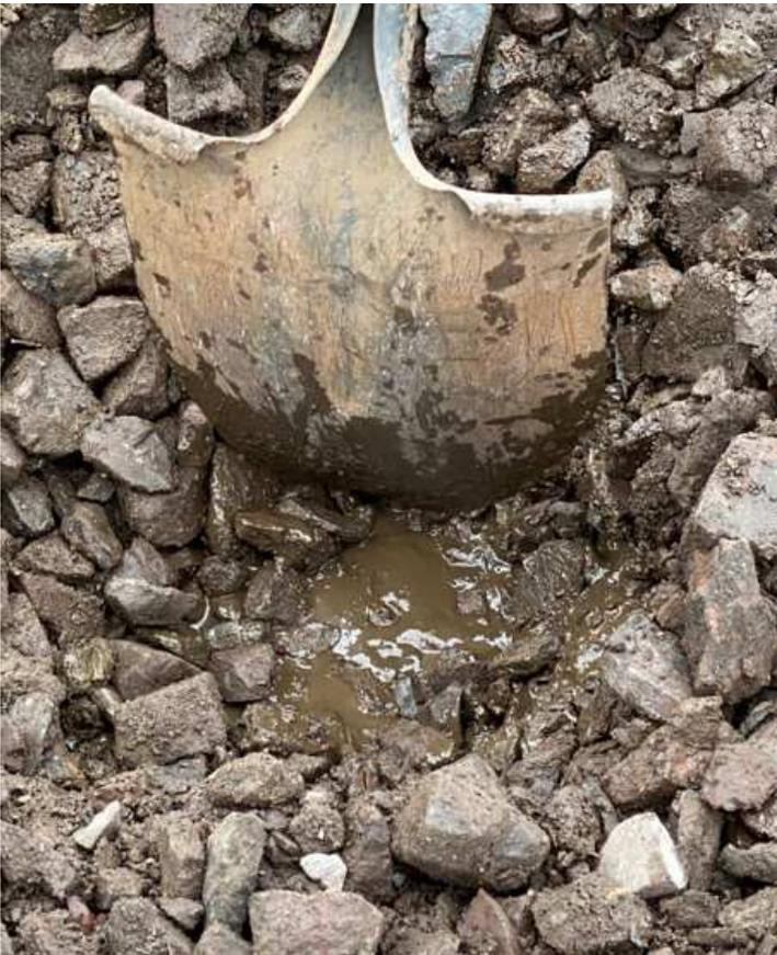
**Fouling was evident in the middle of the roadbed at approximately 1ft beneath the sleeper.**
