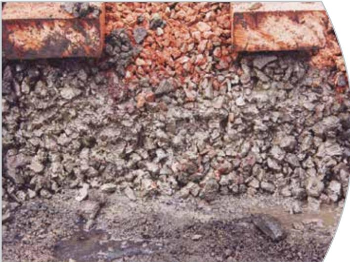
Slurry is shown pumping its way up through the ballast
