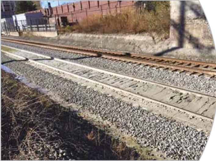
Movement of slurry (fine-grain material and water) from subgrade to track level
