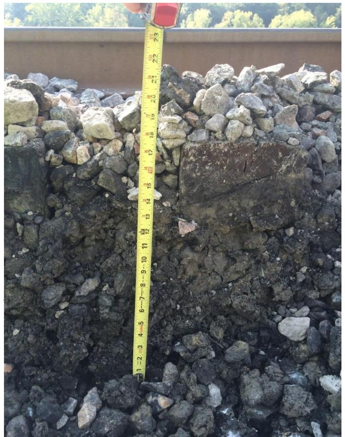
The initial test sections were installed in 2014, and by December 2016, several mud boils had developed in the low-side shoulder of the track which were then removed by an excavator. Photos were then taken during an inspection in April 2017 that showed the clean crib ballast.
